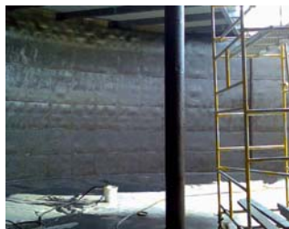
Liquid Rubber used to seal & protect a large volume water tank
